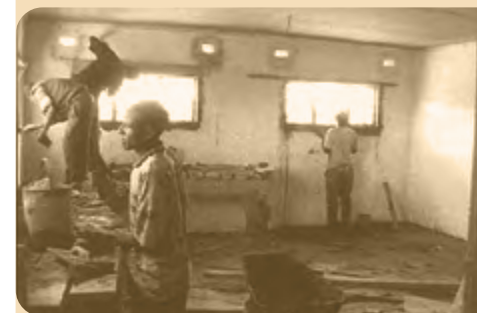
Interior finishing in progress
